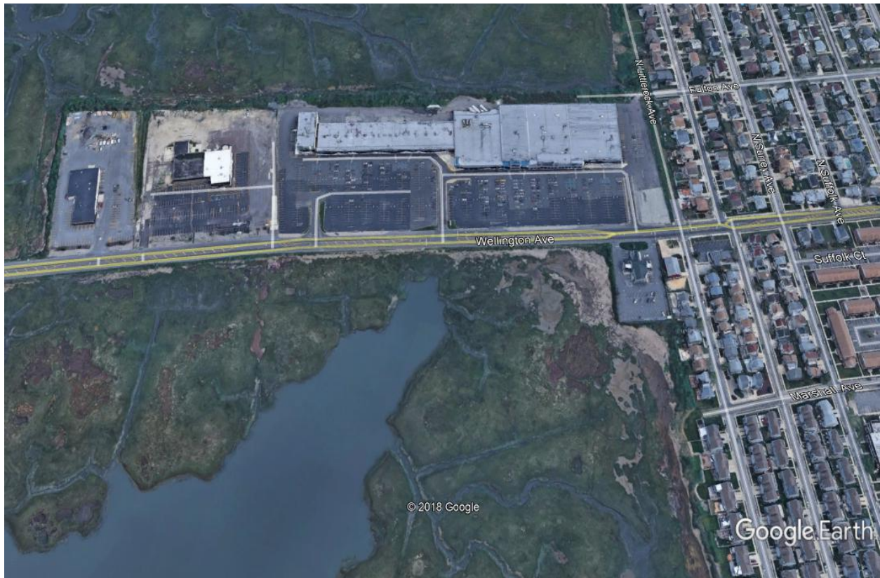
Figure 3 - Aerial of Ventnor Plaza Site
