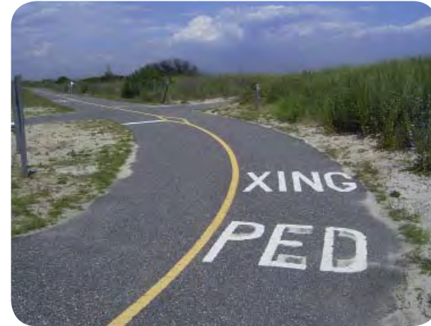
SHARED USE PATH IN HIGHLANDS, NJ
