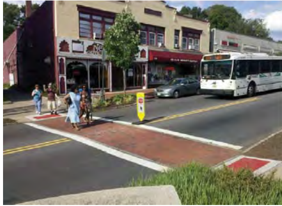
TEXTURED CROSSWALK WITH IN-STREET PEDESTRIAN CROSSING SIGN
