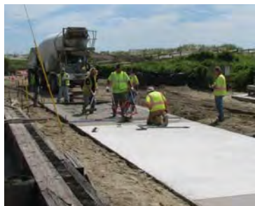
BEACH PATH CONSTRUCTION IN N. WILDWOOD
