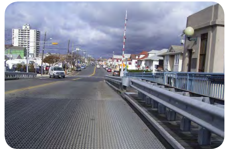
DORSET AVENUE BRIDGE
